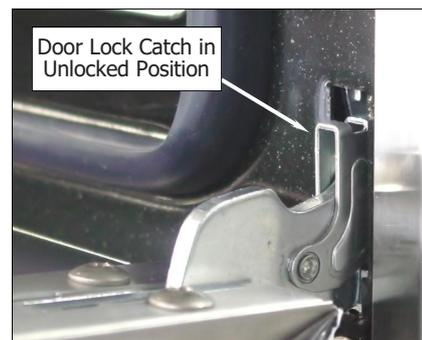
**NOTE:** Check that both Door Lock Catches are in the 'Un-Locked' position before closing the door.
