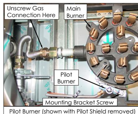
8. Refit the Pilot Shield to the Pilot Bracket, (this is a push-fit onto the pilot bracket).
