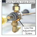
The 'Low Fire Screw' should be sealed with coloured paint on completion of the low fire adjustment.
